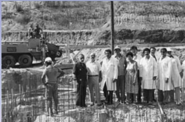
School faculty inspect the foundations of the new edifice.
